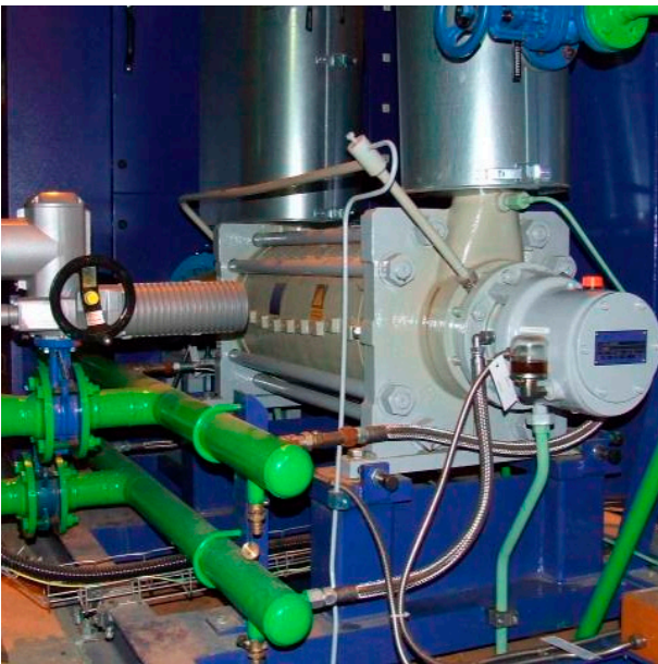
Auxiliary feed-water pump CTD 3.1, Coal-Fired Power Plant Nováky (Slovakia). Unit consists of pump, gearbox and diesel engine.
